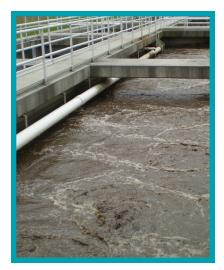
To meet a new year-around total-phosphorus limit at the 6.1 MGD Westfield wastewater treatment facility, the first third of the plug flow aeration tanks are operated as fermentation tanks. To keep the tanks mixed, modifications have been made to the fine bubble aeration disks. The membrane covers have been removed on over 95% of the disks and the air ports plugged with stainless steel screws. The remaining disks have been cut so that large bubbles of air escape and mix the tank contents.
