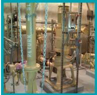
The air flow to the first two passes of the four pass 0.4 MGD extended aeration facility was reduced to create a habitat for nitrate reduction. The return activated sludge pumps are operated at 200% of the influent flow rate to bring nitrate rich flow into the pre-anoxic tank.
