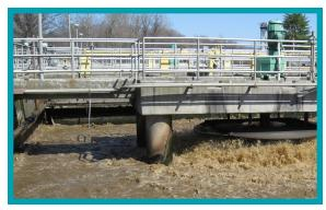
A 2008 BioWin modeling study concluded "the existing facility has half of the necessary volume at the current flows... to consistently achieve [8 mg/L effluent] nitrogen..." A \$61 million dollar facility upgrade to Amherst's 7.2 MGD mechanical aeration facility was found necessary.
