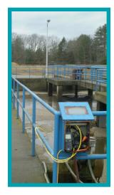
After a decade of study, a report recommending a \$45 million replacement of Plainfield's 1.0 and 0.5 MGD activated sludge plants with a new sequencing batch reactor (SBR) was prepared by the Town's former consultant. A \$10,000 investment in monitoring equipment and ongoing process support by CleanWaterOps demonstrated that the two plants could reliably meet new nitrogen and phosphorus limits, negating the need for their replacement.
